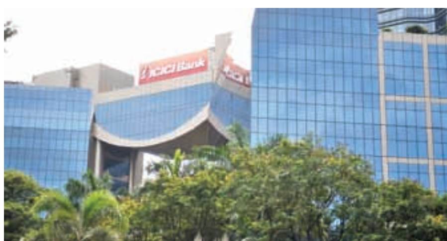
ICICI Bank building in Mumbai.
