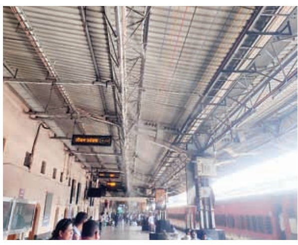
Misting system installed at Raipur station becomes operational.
