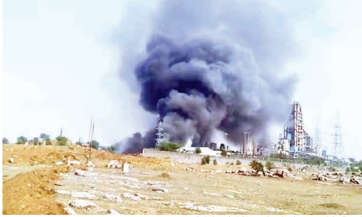
Fire broke out in Shri Cement plant when the waste was being disposed.
