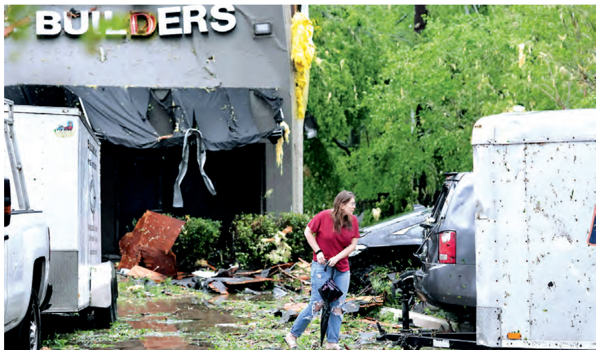
A woman walks amidst rubble of a heavily damaged building in the aftermath of severe storms that swept through the region in Slidell, La.
