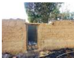
Remains of the house which caught fire.
