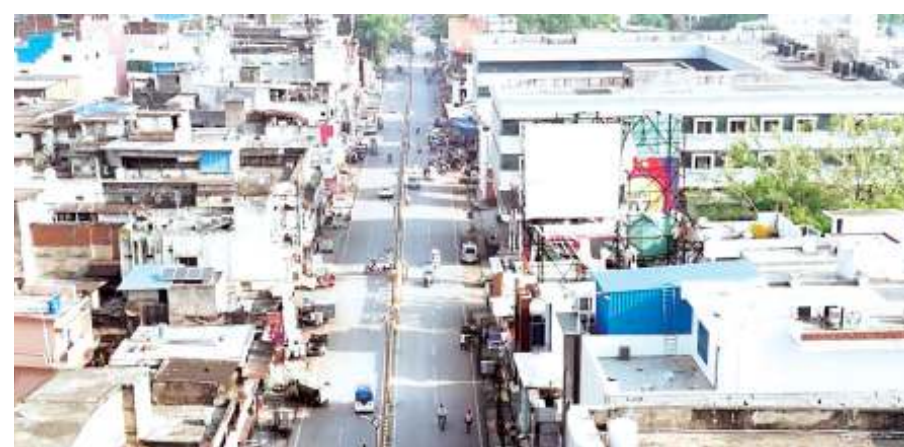
Raipur Smart City Limited eliminated electric wires from Malviya Road.
