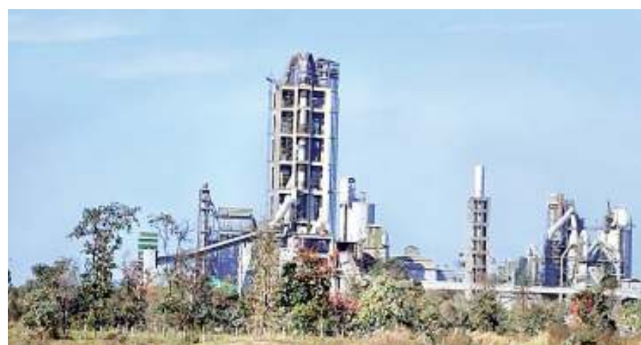
At least six persons were burnt in a major mishap in mines of Ambuja Cement Plant on Friday.
