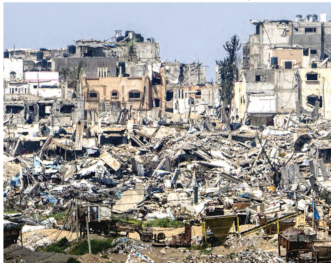
Destroyed buildings stand inside Gaza Strip, as seen from southern Israel, Tuesday, March 19.
