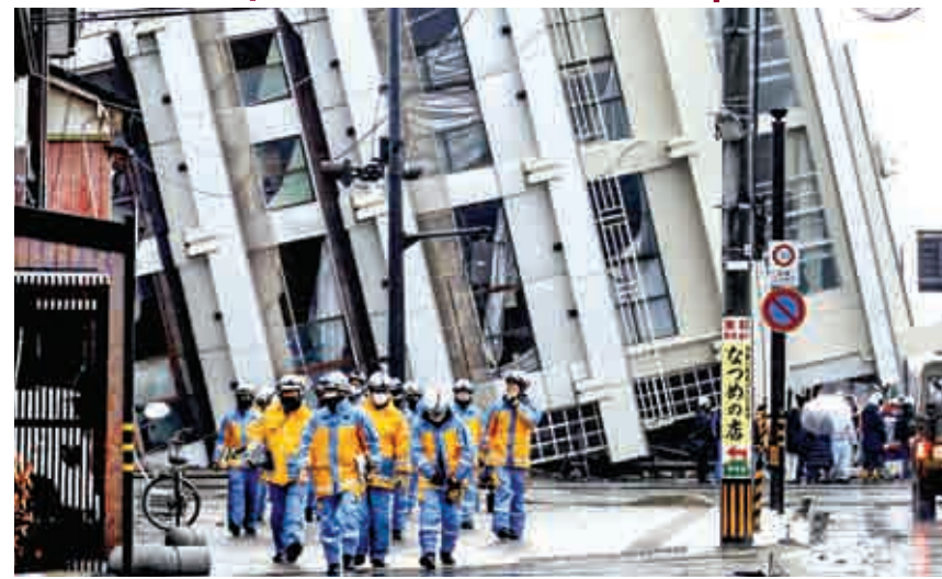
Firefighters walk near a fallen building following earthquakes in Wajima, Ishikawa prefecture, Japan Wednesday, Jan. 3. A series of powerful earthquakes that hit western Japan left multiple people dead Wednesday, as rescue workers fought to save those feared trapped under the rubble of collapsed buildings.
