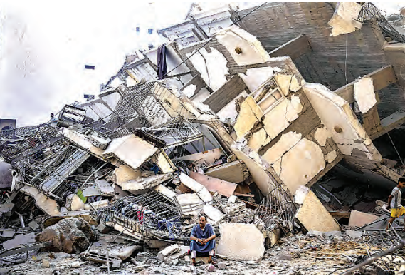
A Palestinian man sits in the rubble of a building after it was struck by an Israeli airstrike, in Gaza City, Sunday.
