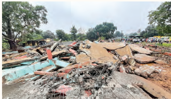
Debris of the collapsed twin tanks
