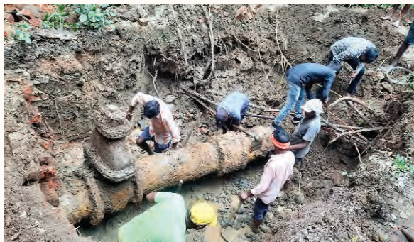
Main line being connected with supply network
