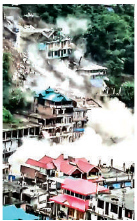
Buildings collapse due to a rain-triggered landslide at Anni town, in Kullu district, Thursday.
