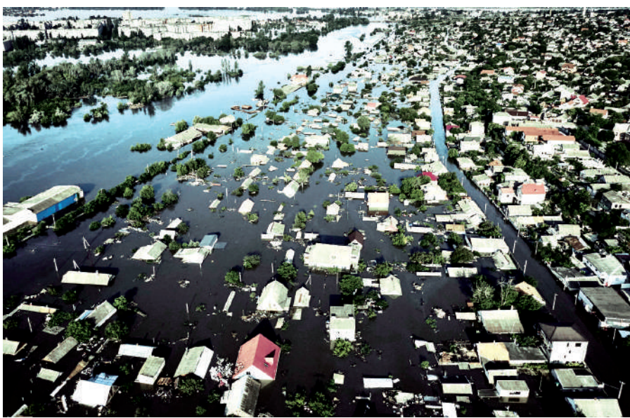
Streets are flooded in Kherson, Ukraine, Wednesday, June 7 after the walls of the Kakhovka dam collapsed. Residents of southern Ukraine, some who spent the night on rooftops, braced for a second day of swelling floodwaters on Wednesday as authorities warned that a Dnieper River dam breach would continue to unleash pent-up waters from a giant reservoir.
