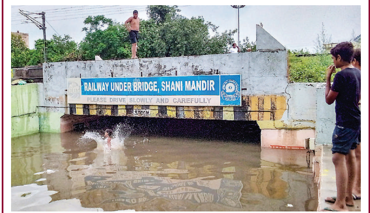
Waterlogged Shani Mandir railway underpass after heavy rainfall in Sonapat, Sunday.
