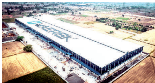
A warehouse of integrated logistics firm A.P. Moller - Maersk in Farrukhnagar.
