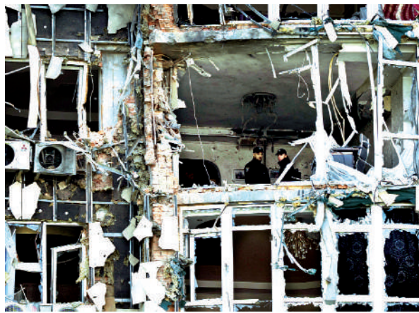
Police inspect an apartment building damaged by a drone, that was shot down during a Russian overnight strike, in Kyiv, Ukraine, Monday.
