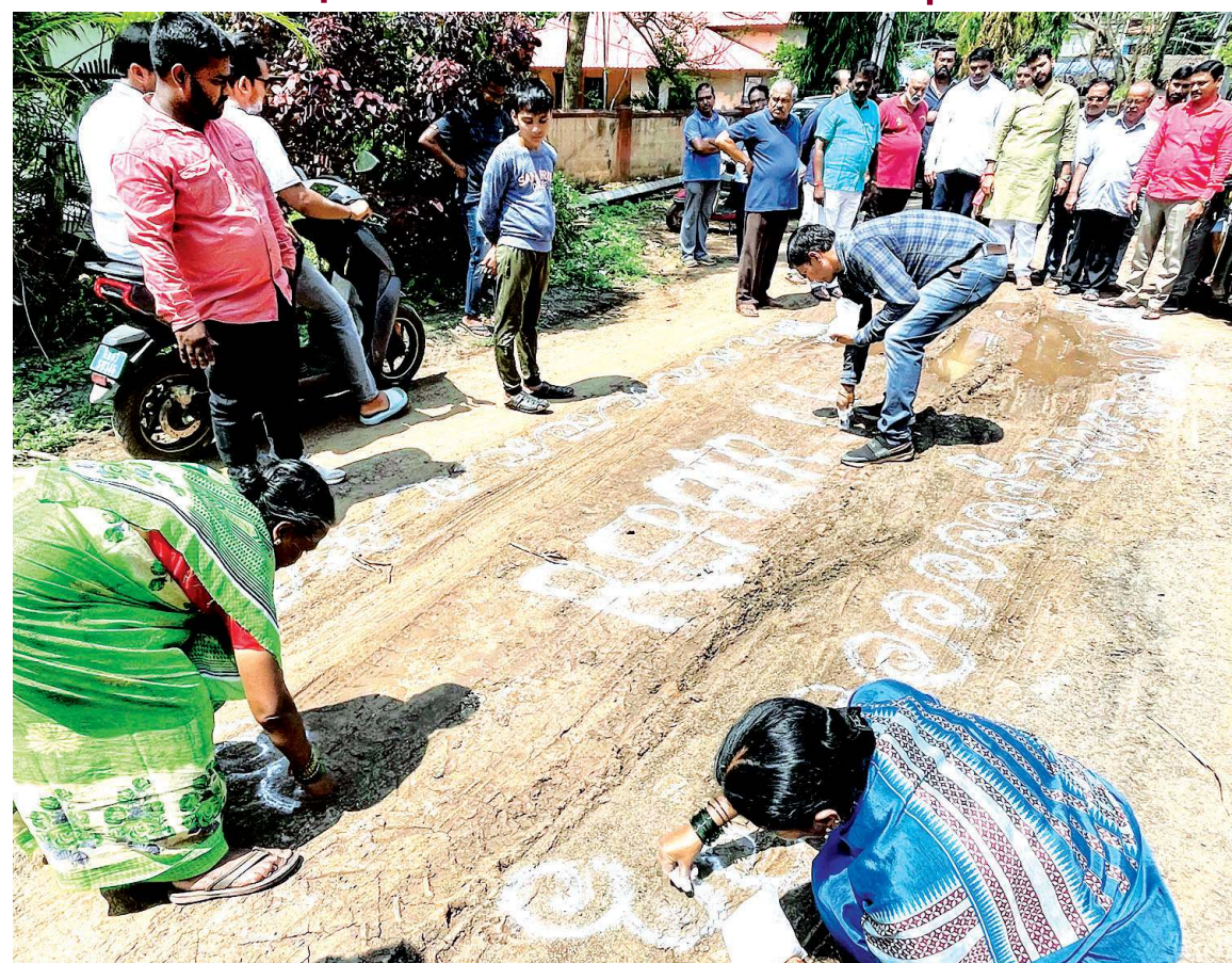
Residents make a rangoli as protest, demanding the repair of damaged roads at Keshwapur, in Hubballi, Karnataka on Wednesday.
