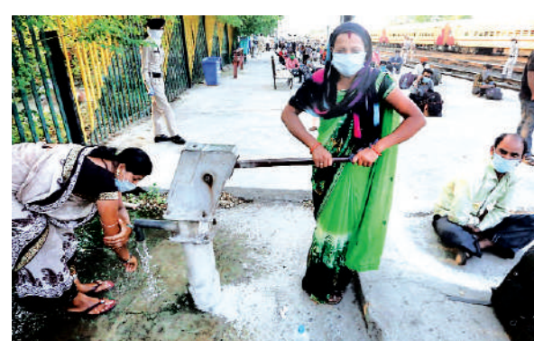
A handpump in Bihar.
