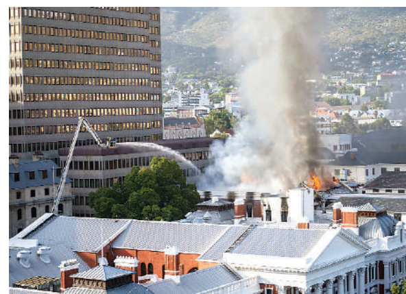
Firemen spray water on flames erupting from a building at Parliament in Cape Town.
